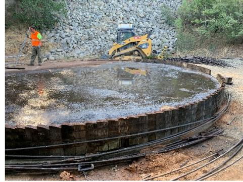
**Magnolia Force Main Replacement** – Work continues on the replacement of wastewater force mains running underneath Dry Creek. Two large pits (bore pits) are very near completion and the sub-contractor specializing in tunneling will begin moving equipment on site next week. With tunneling equipment arriving, the schedule anticipates boring under Dry Creek to begin the second week of September.
